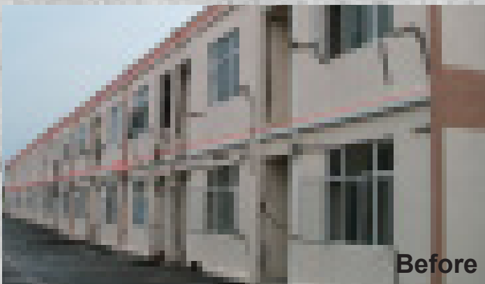
Uplifting to correct the settlement tilt of the building will require synchronised jacking of the underpinning piles prior to pile locked off.
